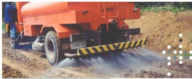
Fig: 4.3 Application of TerraZyme to subgrade
