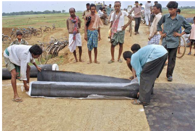
Fig:3.1: Use of Jute Geo-textile
