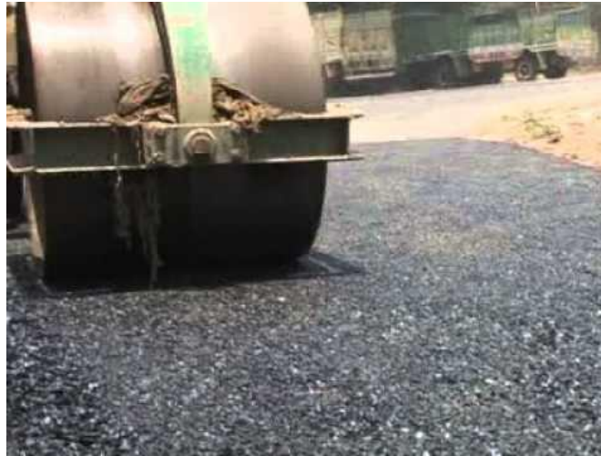
Fig:3.2: Use of Waste Plastic Blended Bitumen
